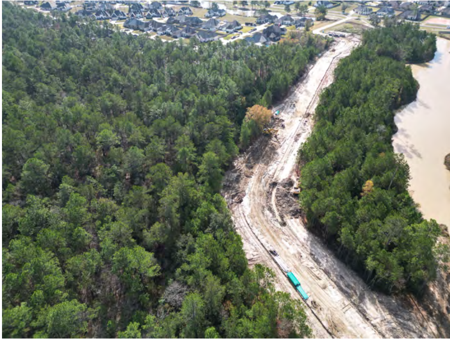
Photo 10: View looking S.
