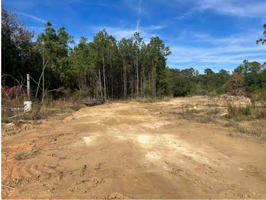
Photo 07: View looking N into new construction area.
