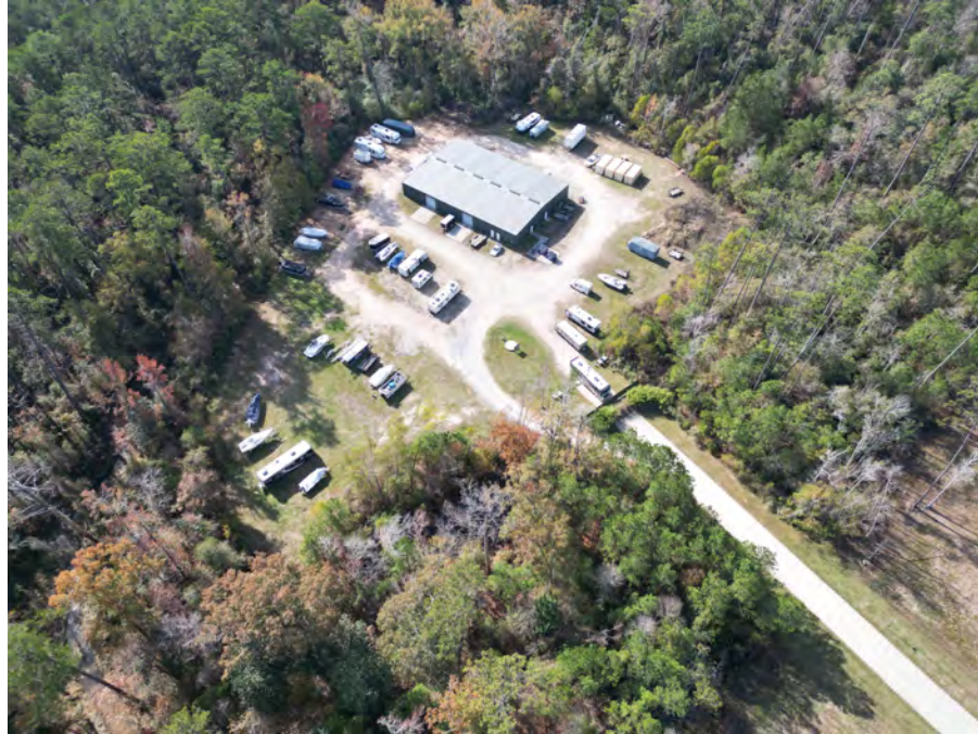
Photo 27: View looking at storage unit facility.
