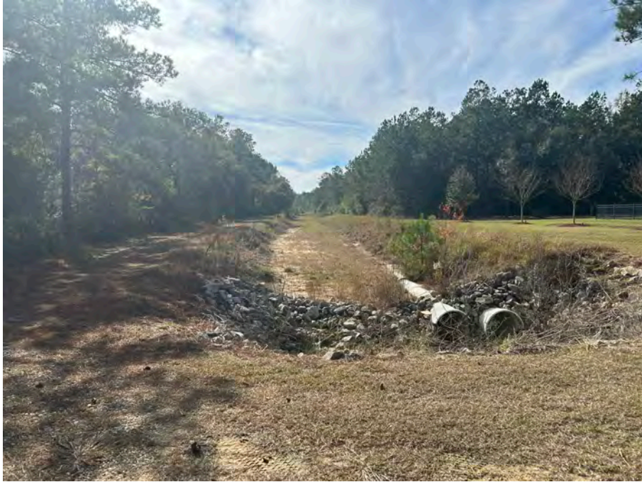
Photo 05: View looking SW along large drainage ditch inside of servitude area.
