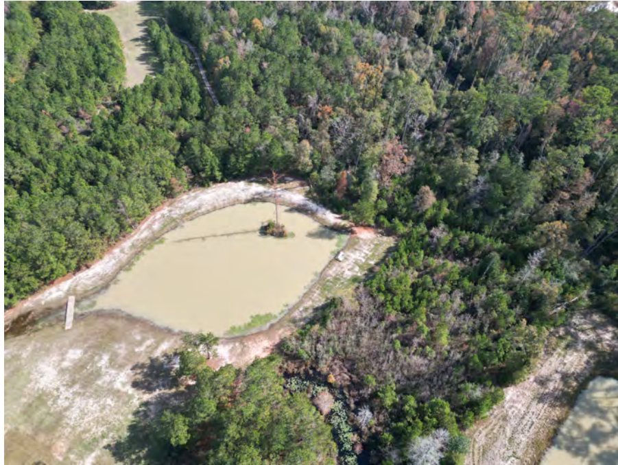
Photo 25: View looking down at previous storm damage at servitude boundary.
