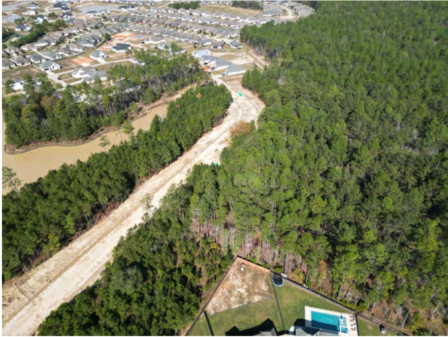
Photo 17: View looking NNW.
